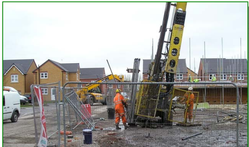
Angled Probe Drilling Beneath Estates Road
